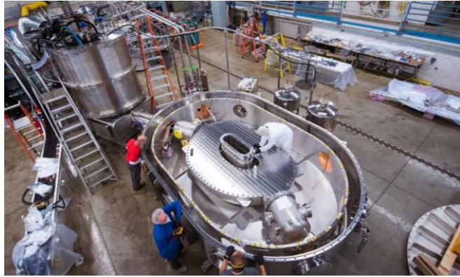
Figure 3: The TFMC being installed into the vacuum cryostat in the TFMC Test Facility at the MIT Plasma Science and Fusion Center.
