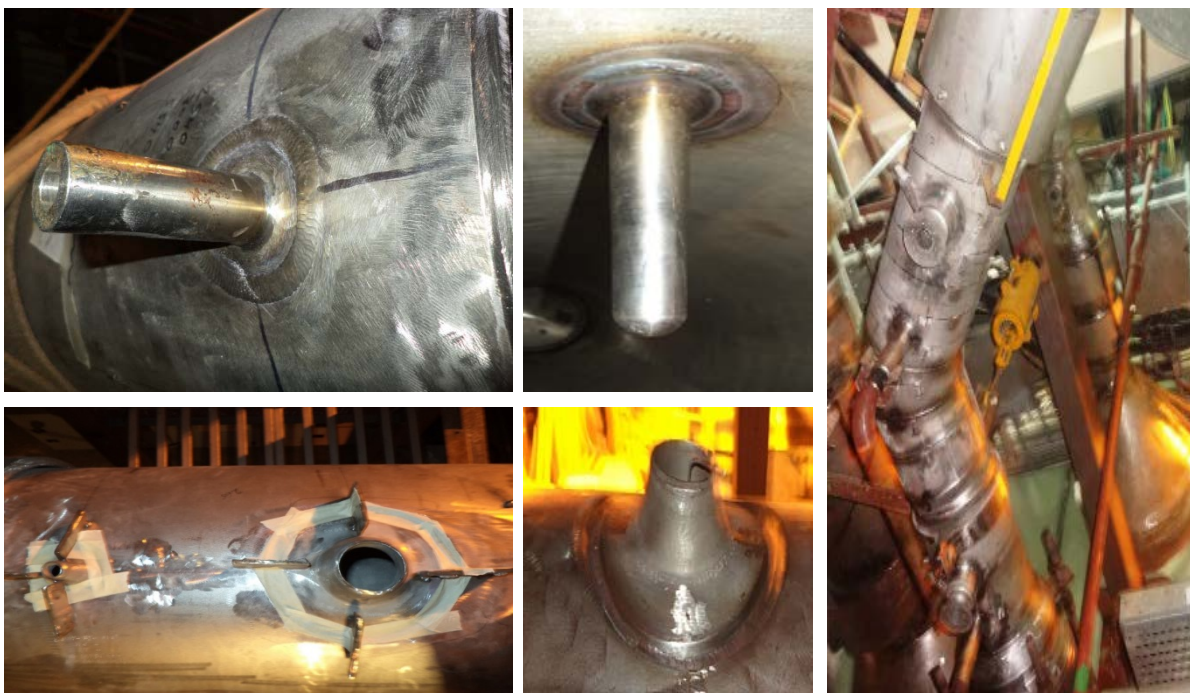
FIG. 4. Thermowell welding, button pull-outs and guard pipe welding
