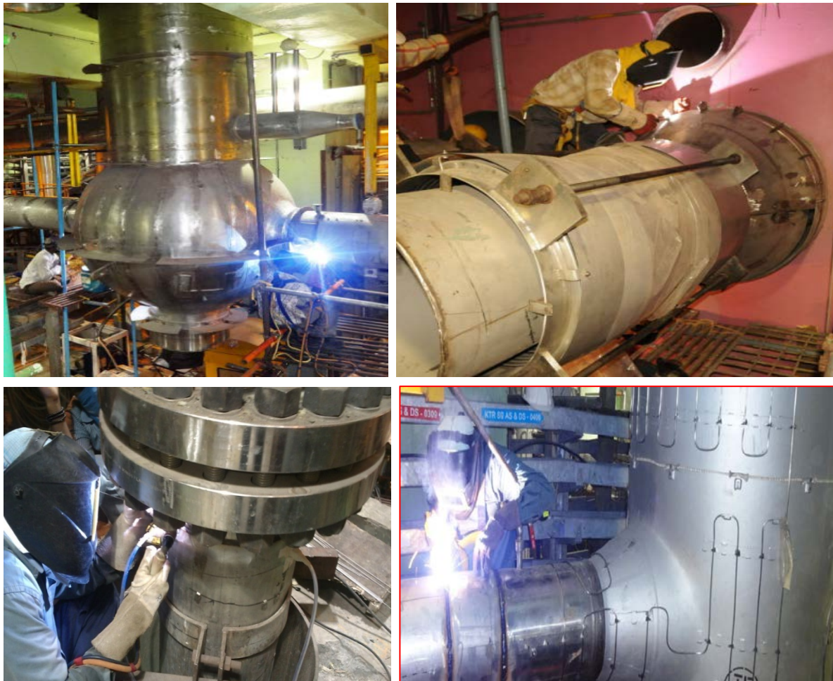
FIG. 3. Sequential and systematic welding of sodium pipe lines at site
