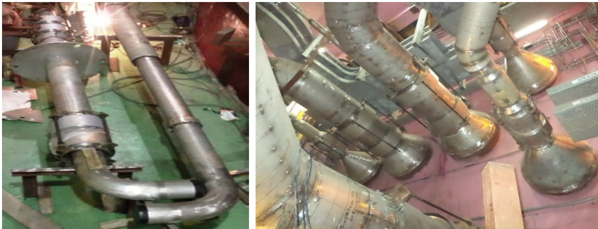
FIG. 6. Hot pipe wall penetrations- fabrication and erection
