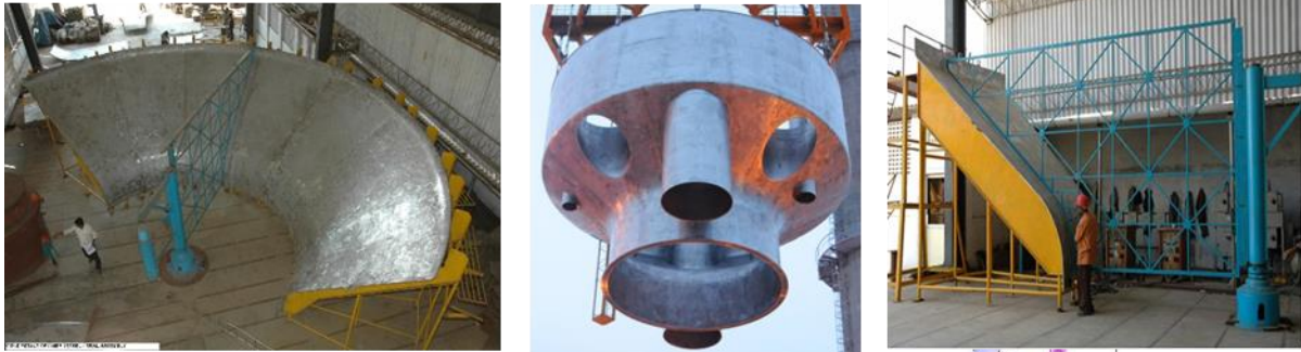
Fig. 6. Stand Pipe Weld on Inner Vessel
