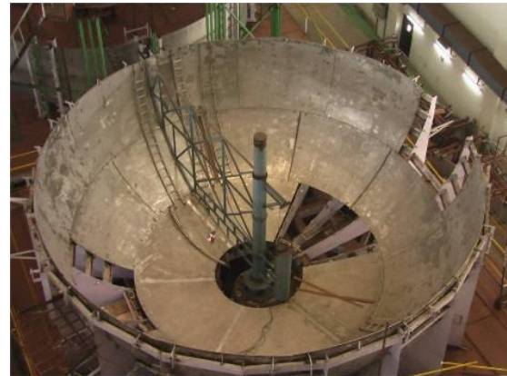
Fig. 3. Safety Vessel Dished End with Swing Arm Gauge
