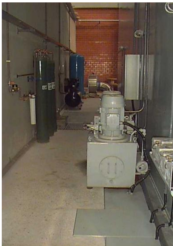
Hydraulic system (tote boxes irradiator)
