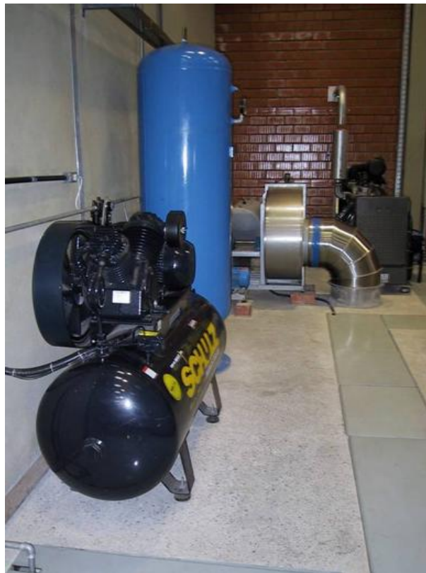
Pneumatic ( ^{60}\text{Co} source racks) and ventilation ( \text{O}_3 ) systems
